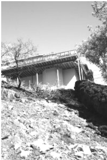
Minimal ground fuels treatment saved 200 houses near Lake Arrowhead
